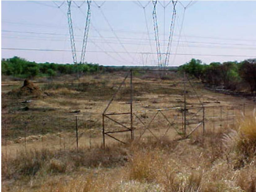
**Figure 3.** A game fence as used on the Matimba-Spitskop 1&2 lines. Note that the top section has been omitted as per the latest 5m game gate design.
